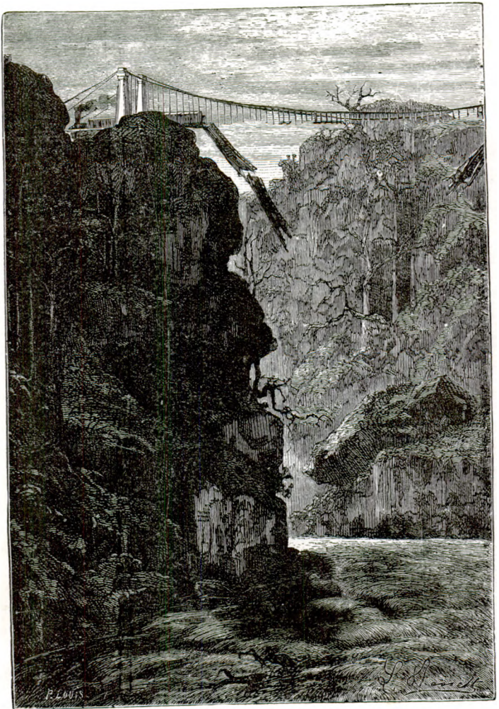
"The bridge, completely ruined, fell with a crash." — Page 241.
